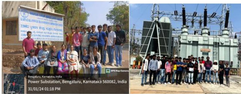
Fig.4 Visit to 220 KV Sub-Station, Somanahalli, Bengaluru
